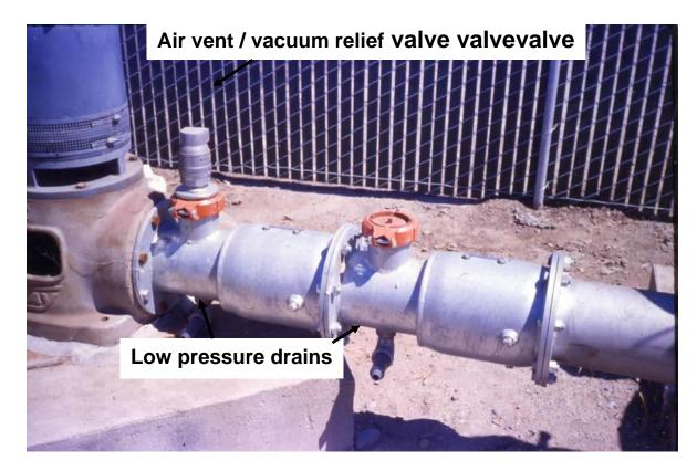
**Figure 17d** Double chemigation check valve protecting a well from backflow contamination. A double check valve is required in some States and is installed for safety redundancy.
