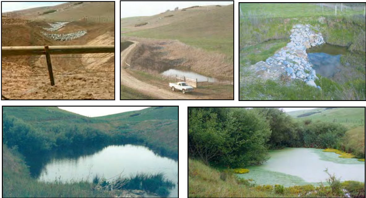
Figure 31: A series of seven small Grade Stabilization Structures were installed in the gully as loose rock checkdams above a Sediment Basin in 1989 with preproject photo (top left), aerial view design (top right), immediately following construction (middle left), the site two years later (middle), checkdam structure functioning as designed (middle right), four years (bottom left), and six years later (bottom right). Designed by Prunuske Chatham and NRCS.
