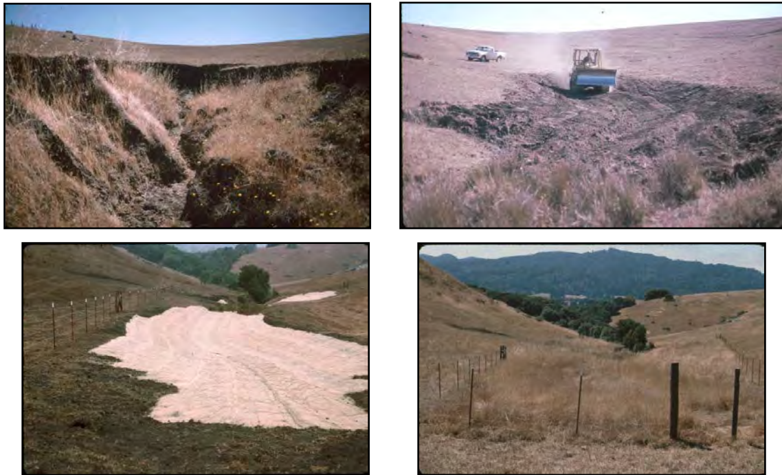
Figure 33: A Grassed Waterway practice installed in Lagunitas Creek Watershed in 1988. Designed by NRCS.
