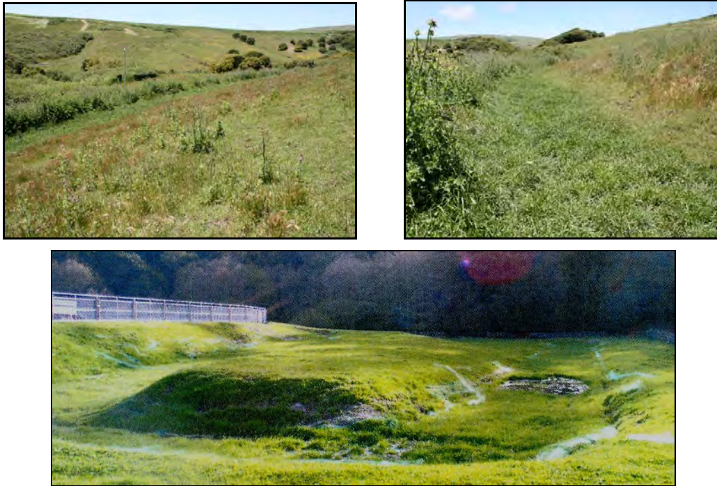
Figure 23: Examples of Filter Strips to treat surface water runoff from corrals depicting an overview of a hillside site with over 400 feet of laminar flow conditions following the contour (top), and a flat bottomland location where the site's treatment distance and laminar flow conditions were maximized (bottom). Designed by NRCS.
