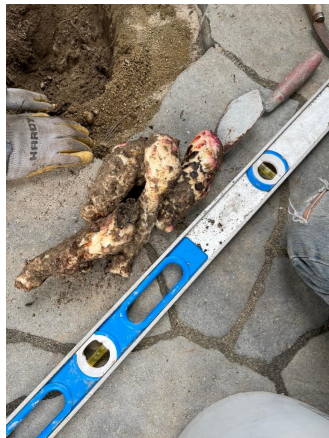
This root pushed up through We dug it out to about 18"
