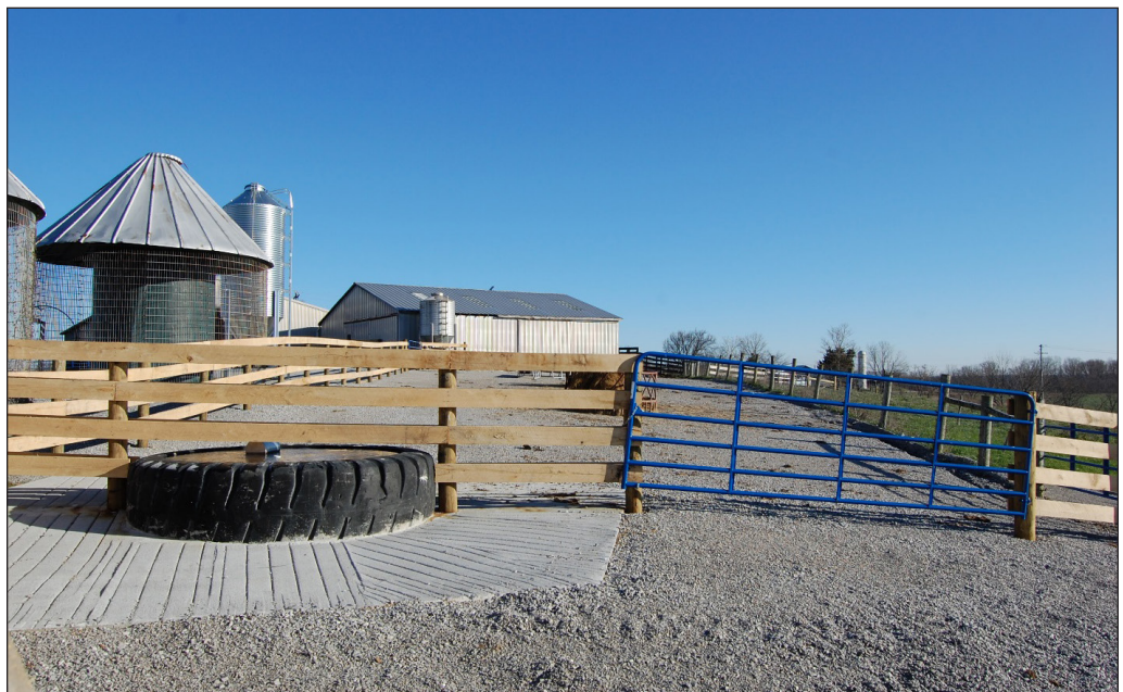
Figure 5. Large volume tire waterer tank installed in heavy-use area. Photo by Lee Moser
