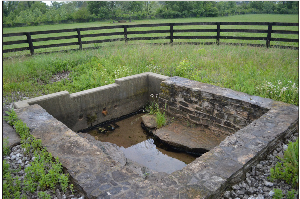
Figure 3. Developing springs can provide producers with an inexpensive, clean water source. Depending on their location, developed springs can be used to deliver water away from sensitive areas by gravity flow. Photo by Amanda Gumbert
