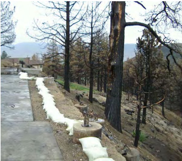
Severely burned trees will not survive.
