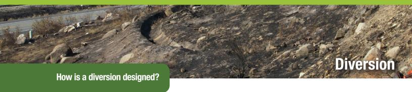
Diversions designed to protect major structures, homes, school buildings and high capacity roads shall have enough capacity for the 100-year frequency 24-hour duration storm.
