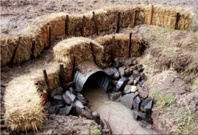
Properly installed and protected culvert.
