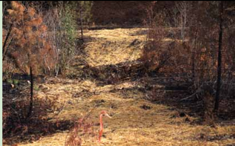
Straw mulch applied to a burned site.
