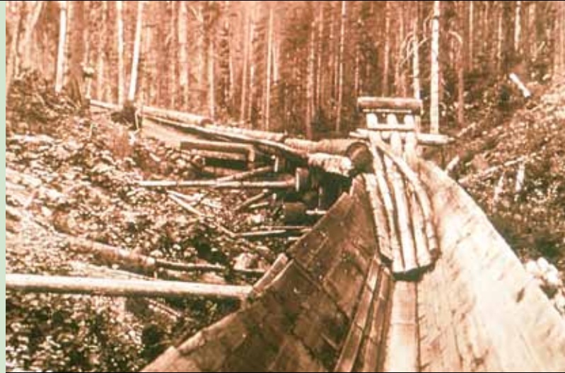
Logs being moved downhill in a flume.
