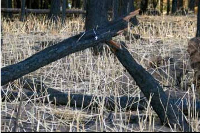
Straw mulch anchored into soil by punching.
