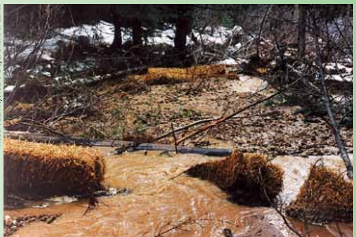
Failed staw bale check dam.
