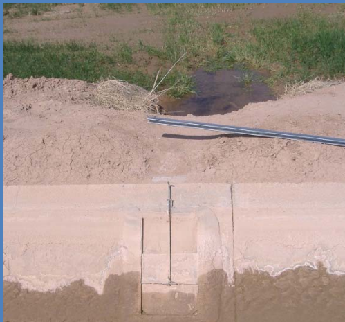
Existing Port Gates
