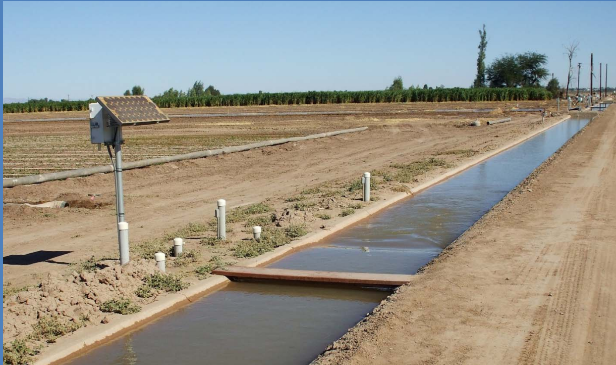
Flow Measurement – Main Control Station
