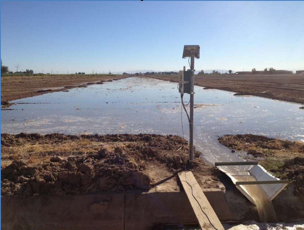
Field Runoff Measurement Station
