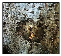
Fig.6 "Watermark" staining (Courtesy of OC Parks)
