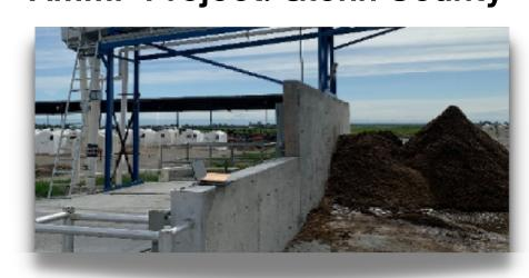
A manure solid separator keeps solids out of the manure pond.
