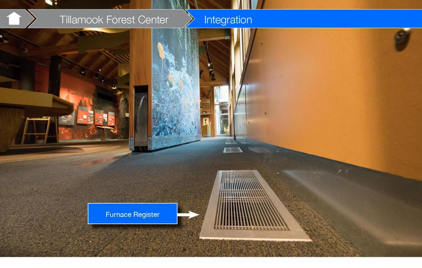
**Integration:** Heat for the main exhibit halls is delivered through forced air registers in the floor (like those found in many homes). Forced air heating systems do double-duty—delivering heat and fresh air.
