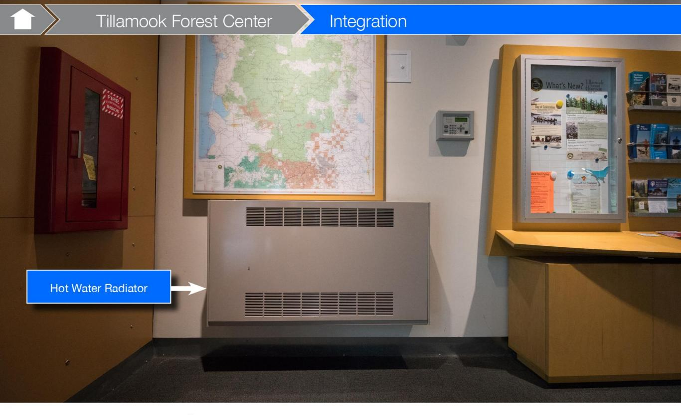
**Integration:** Offices, rest rooms, and the entry area (above) are heated with hot water radiators like this one. The many independently controlled zones throughout the building provide flexibility to deliver heat only where it is needed. On days when the Center is closed to the public, individual offices can be heated without having to heat the entire building.
