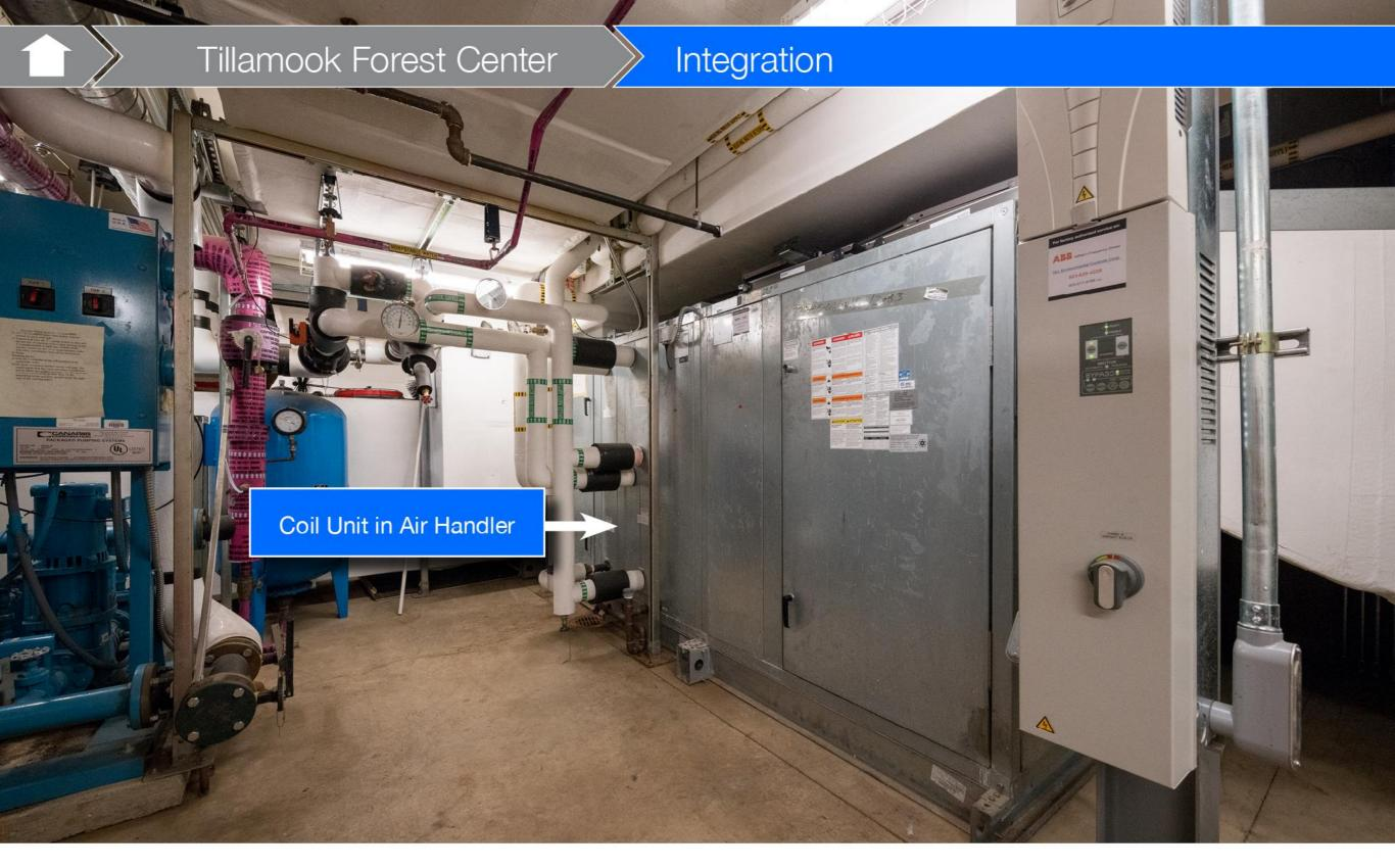
**Integration:** The hot water distribution loop from the biomass boiler integrates with the building's domestic hot water (DWH) system through these two flat plate heat exchangers. If your building will have a forced-air heating system, be sure to have enough room for an additional heating coil that can connect to a future biomass system.
