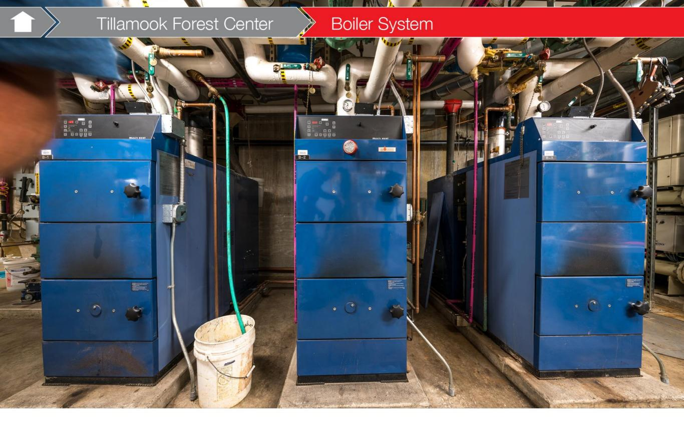
**Boiler System:** approximately 280 sq. ft. (20' x 14') of the 1,500-square foot mechanical equipment room is dedicated to the biomass boiler system. The system is made up of three TARM 136,500 Btu/h wood pellet boilers. Each boiler has an internal pellet storage bin that is semi-automatically filled from the large pellet silo outside.
