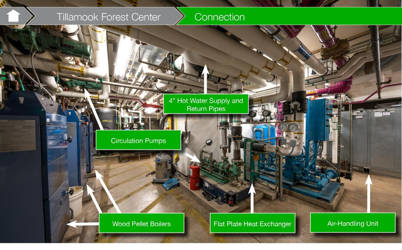
**Connection:** Heat is delivered to the building from the boilers using a combination of forced-air (like a furnace in a typical home) and hydronic (hot water loop) systems. A flat plate heat exchanger (center of diagram) is used to isolate the boiler water from the hydronic water loop that goes both to the fan coil unit inside the air handling unit. The three biomass boilers are the only source of heat in the building. There is no backup heat for the building.
