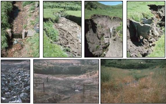
**Figure 32:** Photo monitoring of a grade stabilization project with functional redwood board checkdams before March 1986 storms (top left 2 photos), following March 1986 storms (top right 2 photos), the emergency repair installed a Lined Waterway with control fencing (bottom left 2 photos), and one year later in June 1987 (bottom right). Designed by NRCS.
