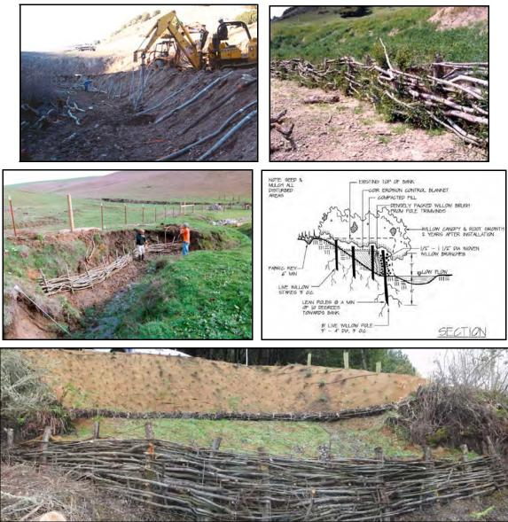
**Figure 36:** An example of the first willow walls constructed in 1990 in the Walker Creek Watershed (top), another later example constructed in 1994 (middle left), a recent design specification (middle right), and a recently constructed willow wall stabilizing the streambank toe below a threatened ranch road with willow fascine and revegetation using native grass seed, sedge/rush plugs, and shrubs in 2008 (bottom). Designs by Prunuske Chatham, Inc.
