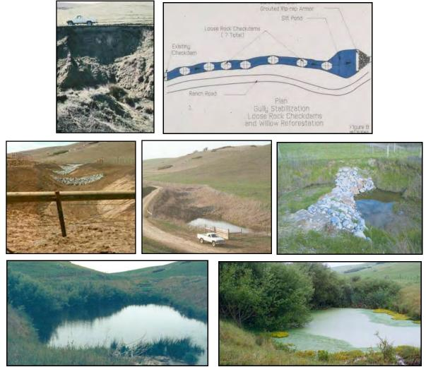
**Figure 31:** A series of seven small Grade Stabilization Structures were installed in the gully as loose rock checkdams above a Sediment Basin in 1989 with preproject photo (top left), aerial view design (top right), immediately following construction (middle left), the site two years later (middle), checkdam structure functioning as designed (middle right), four years (bottom left), and six years later (bottom right). Designed by Prunuske Chatham and NRCS.
