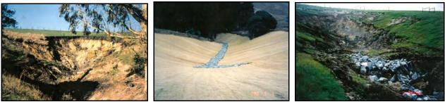
**Figure 34:** An eroding gully pre-project (left), after implementation of Lined Waterway and other practices in 1992 (middle), and four years later the site had unraveled (right).
