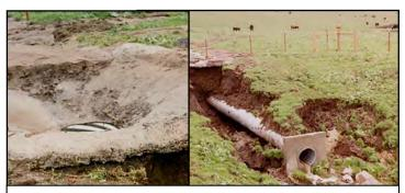
Sediment plugged inlet caused failure of Water Control Structure.
