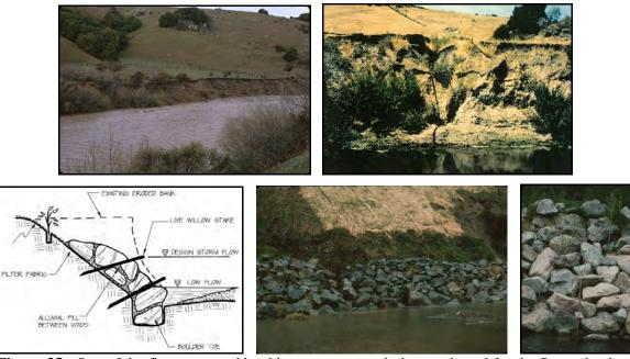
**Figure 35:** One of the first vegetated boulder revetment techniques adapted for the Streambank Stabilization practice at "one of the worst actively eroding streambanks" in Marin County before the project in 1985 (top), practice design and following installation with willow sprouts barely visible (bottom). Designed by Prunuske Chatham, Inc.
