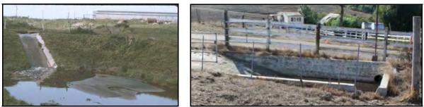
**Figure 29:** Examples of Sediment Basins depicting a large-scale design constructed in the 1980s (left), and a smaller version with a paved access ramp to facilitate maintenance built in 2005 (right).
