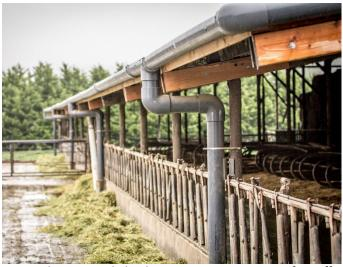
Barn with gutter and plumbing system to capture roof runoff for storage and later use.
