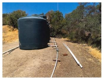
Four 3,000 gallon tanks and plumbing that form a small above ground storage system. This system can store hauled water and is also connected to on-site water sources for storage.
