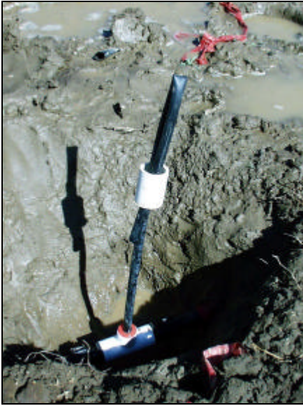
Figure 1. T-port installed in buried drip line with injection access tube.
