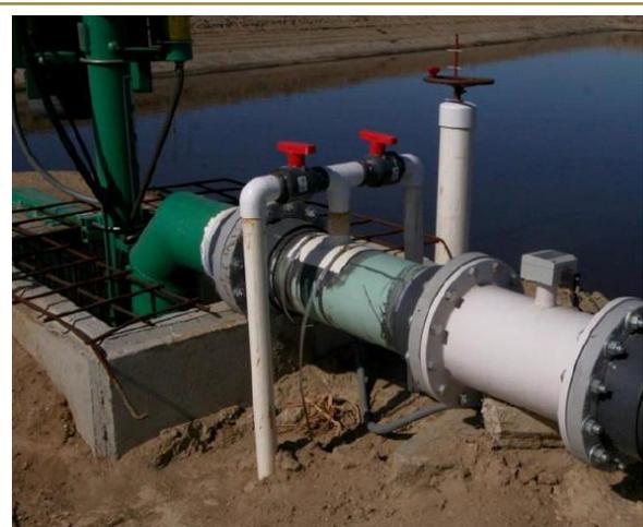
A single pump and metering run serves two adjacent ponds in this system. The pump bypass (red handles) relieves excess pressure on the pump by diverting a portion of the flow to either of two ponds, and can also serve as a way to adjust the application rate of the lagoon water.
