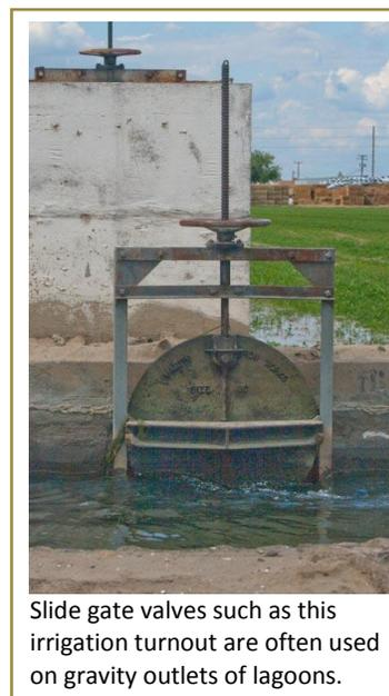
Adjusting the rate from a pond with a gravity flow system can be easier if the valve is a line gate or butterfly valve instead of a slide gate because the diameter of the pipe and valve is usually smaller than is typical with a side gate and the amount of play in the wheel in many cases is less. However, since the pipe diameter is smaller, there may be some limitation on how low a flow rate can be maintained because too small an opening may result in plugging of the valve or outlet pipeline.
