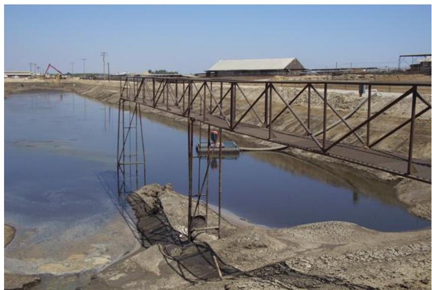
Valves in gravity systems are often accessed from a catwalk. If this valve is used for throttling, it will likely need frequent adjustments. Make certain that the valve can be accessed safely, especially in the dark. This pond has outlets at different depths in the pond, making it possible to adjust the amount of solids in the material being applied.
