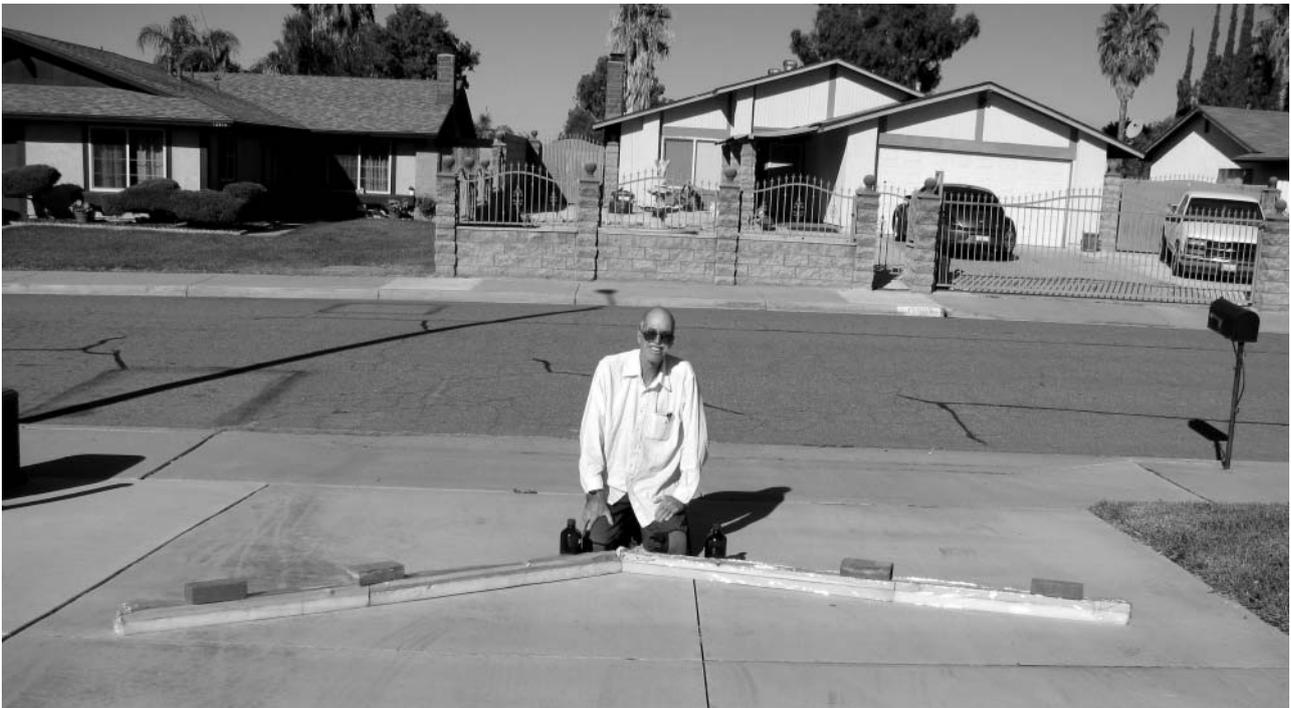
**Figure 1.** Photo of the water dam on a driveway in Riverside, CA. Each side of the dam consists of two 2 × 4s joined with a metal bracket and each half of the dam is attached to a hinge in the middle.
