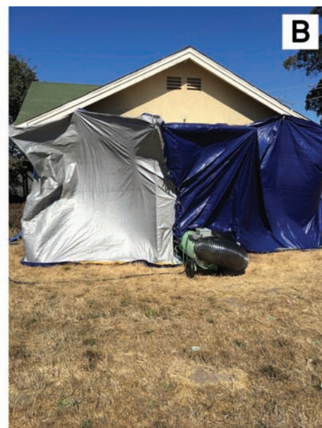
Fig. 2. ‘Villa Termiti’, the experimental structure used in the current study. (A) The south- and west-facing walls of the test structure before beginning treatment. (B) The south wall of the structure during the heat treatment, showing tarpaulins and a heater.
